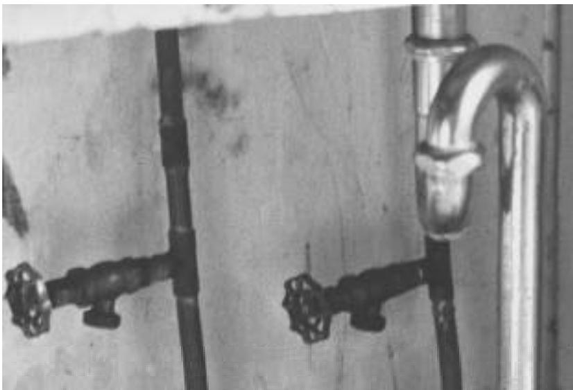
An S-trap that can cause self-siphonage and loss of the water seal. All such traps should be replaced.
