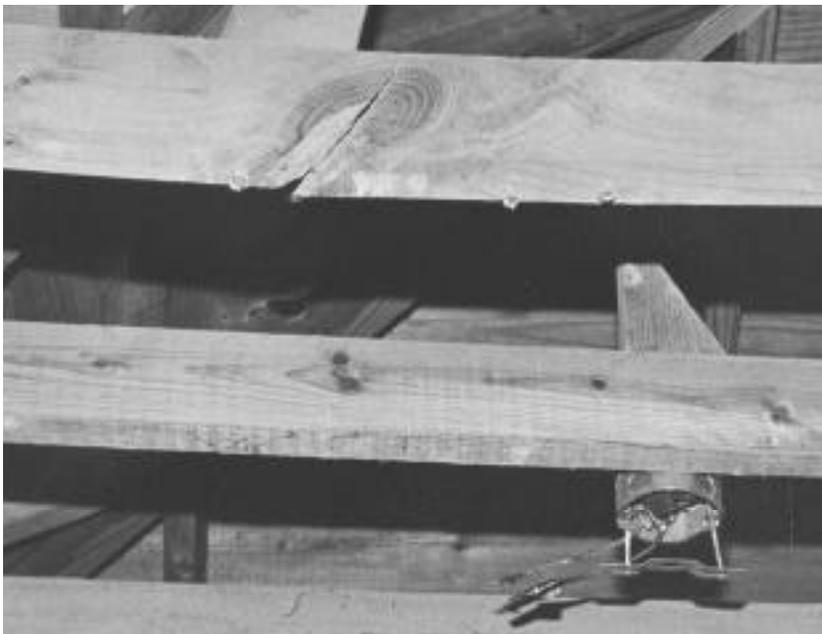
A split ceiling joist or trust chord can be easily repaired by propping it back in place and attaching new structural pieces to each side.
