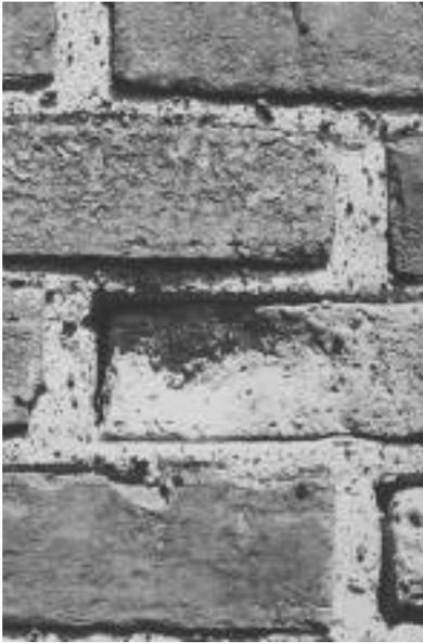
The brick shown here is highly spalled from the effects of excessive moisture penetration and subsequent freezing. The damage cannot be repaired, although individual bricks can be replaced and the mortar pointed. The new mortar should be of the same composition as the old.
