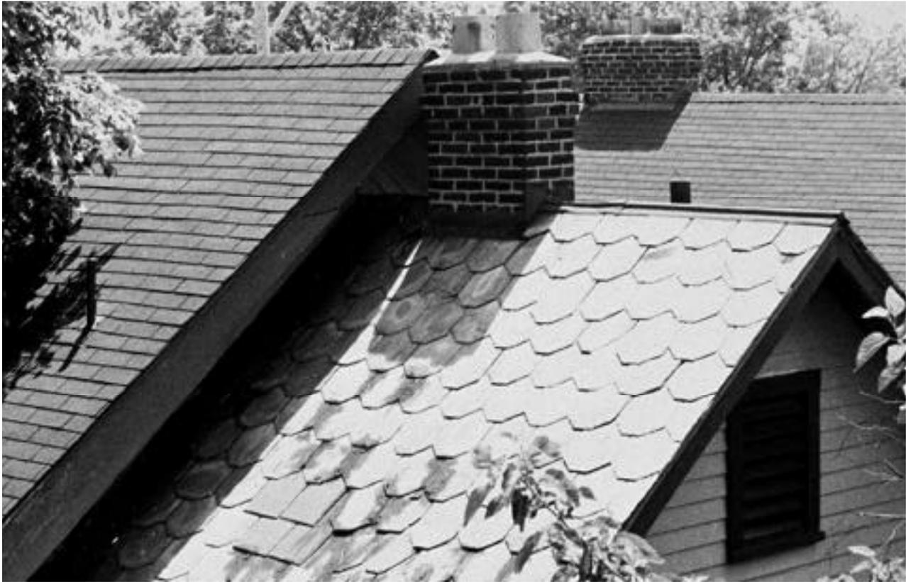
*This slate roof should be carefully investigated since it has a makeshift repair. Other problems include the chimney, which is too low, and the vent pipe, which is too narrow.*
