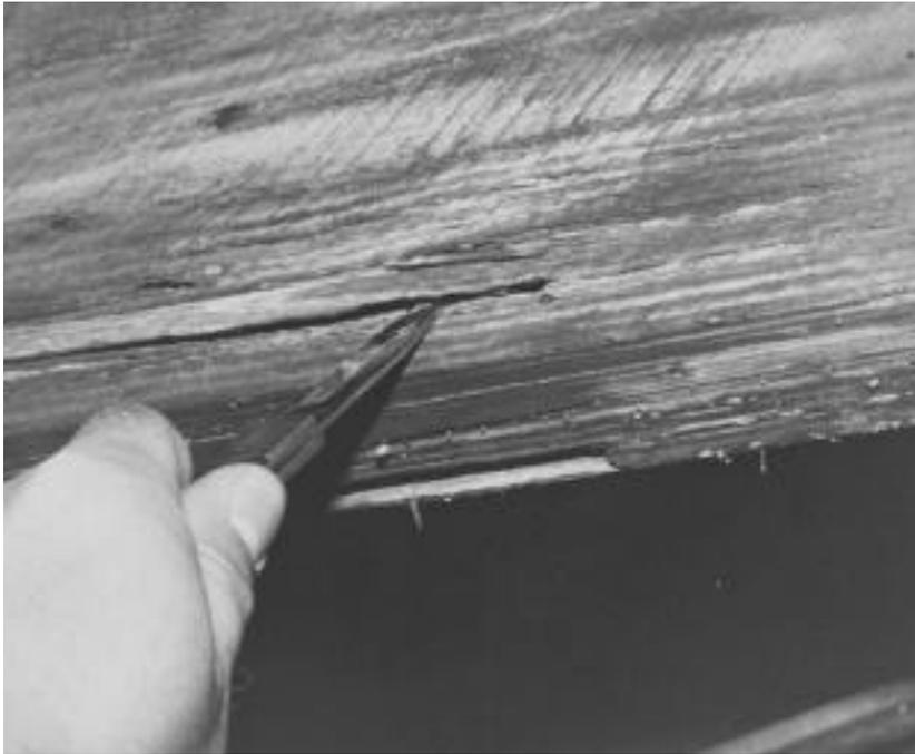
*Termite infestation is most common in basements and crawl spaces, particularly near foundation walls. Probe all suspect areas thoroughly.*
