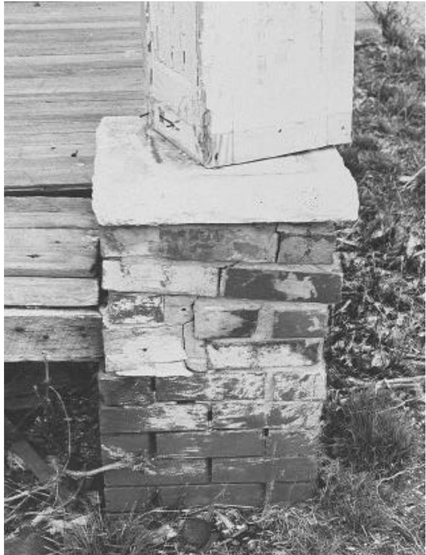
*This pier has been overstressed by movement of the porch and column. The entire assembly should be rebuilt.*
