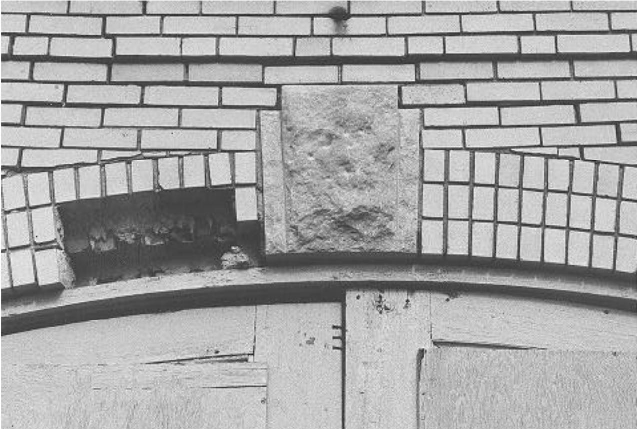
Despite the loss of masonry, this arch is intact and can be repaired with matching bricks.
