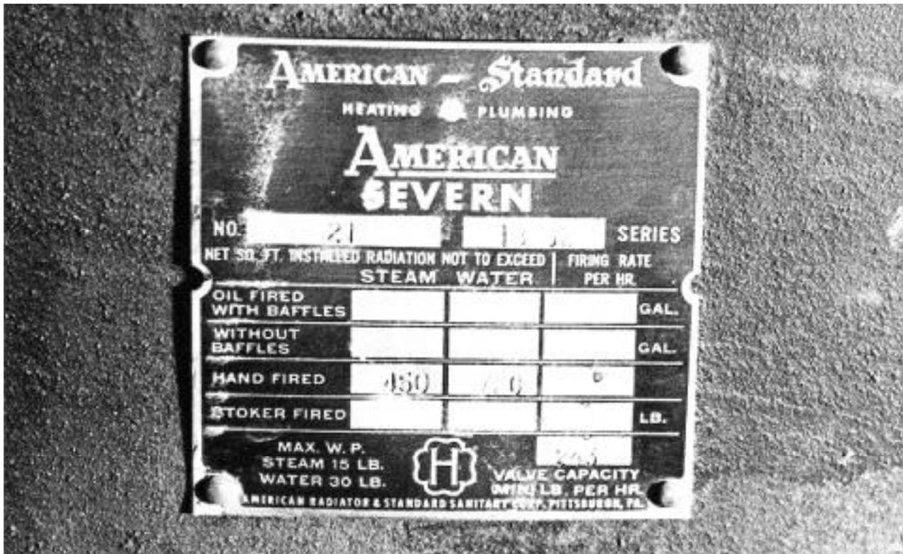
Record all pertinent information from the manufacturer's data plates on HVAC equipment. It will be useful in assessing the equipment's capacity later.
