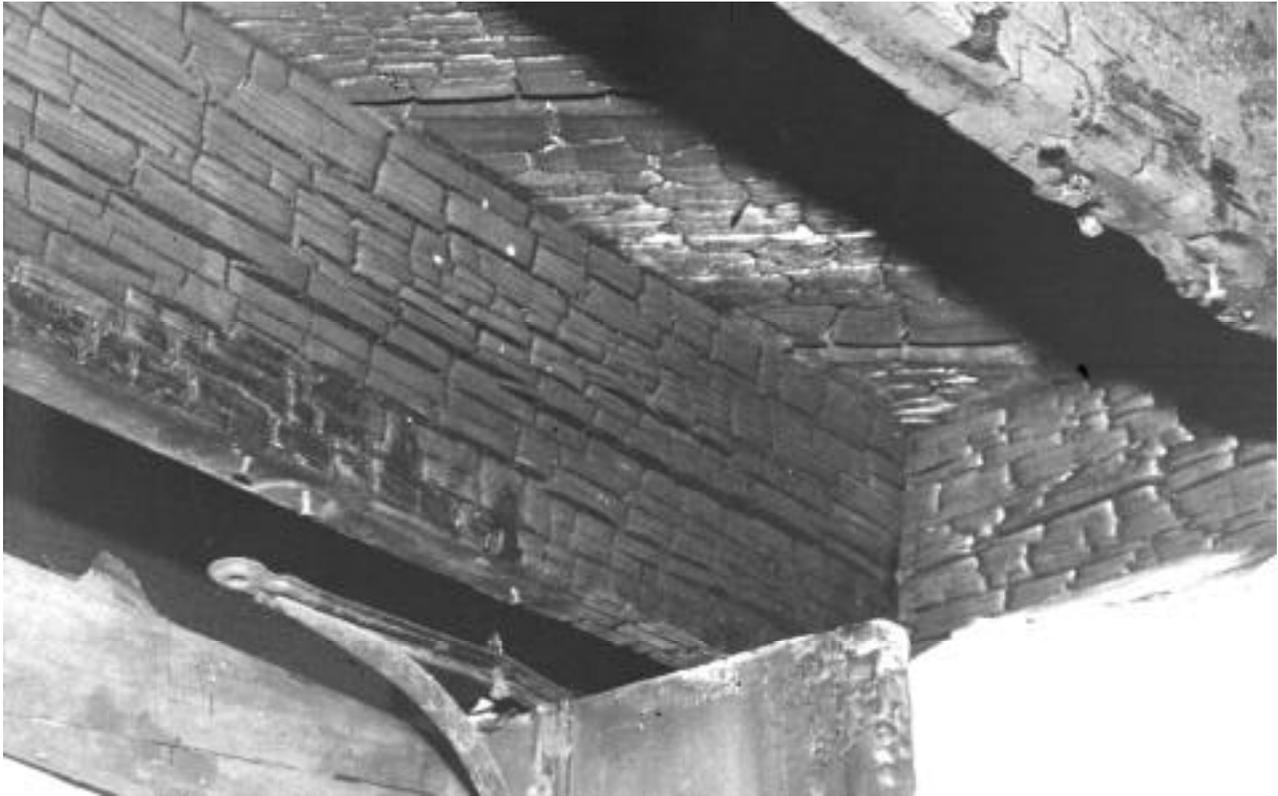
*This fire-damaged wood should be carefully probed to determine the extent of charring. In this case, the wood was replaced.*
