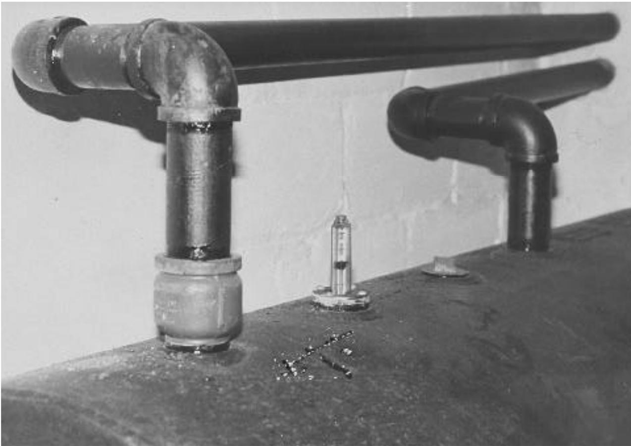
Look for signs of corrosion around and within oil storage tanks and check the operation of the oil level gauge. Use a dipstick to check for signs of condensation in the tank.
